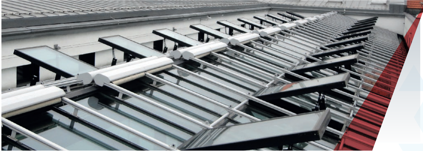
This is how the implementation of smoke dampers for installation in roofs and skylights looks like.
